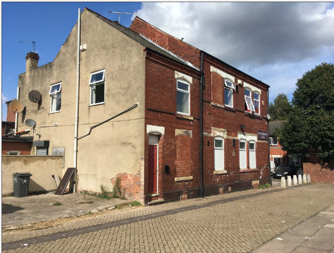
Photo 2 – Application Site: Elevation at Glen Field Avenue
