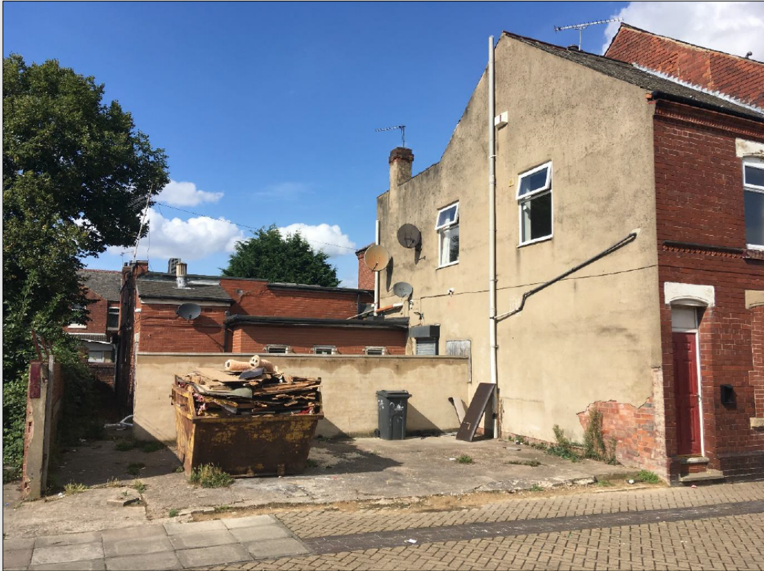
Photo 3 – Application Site: rear yard, including parking area (for flats above) and access for deliveries
