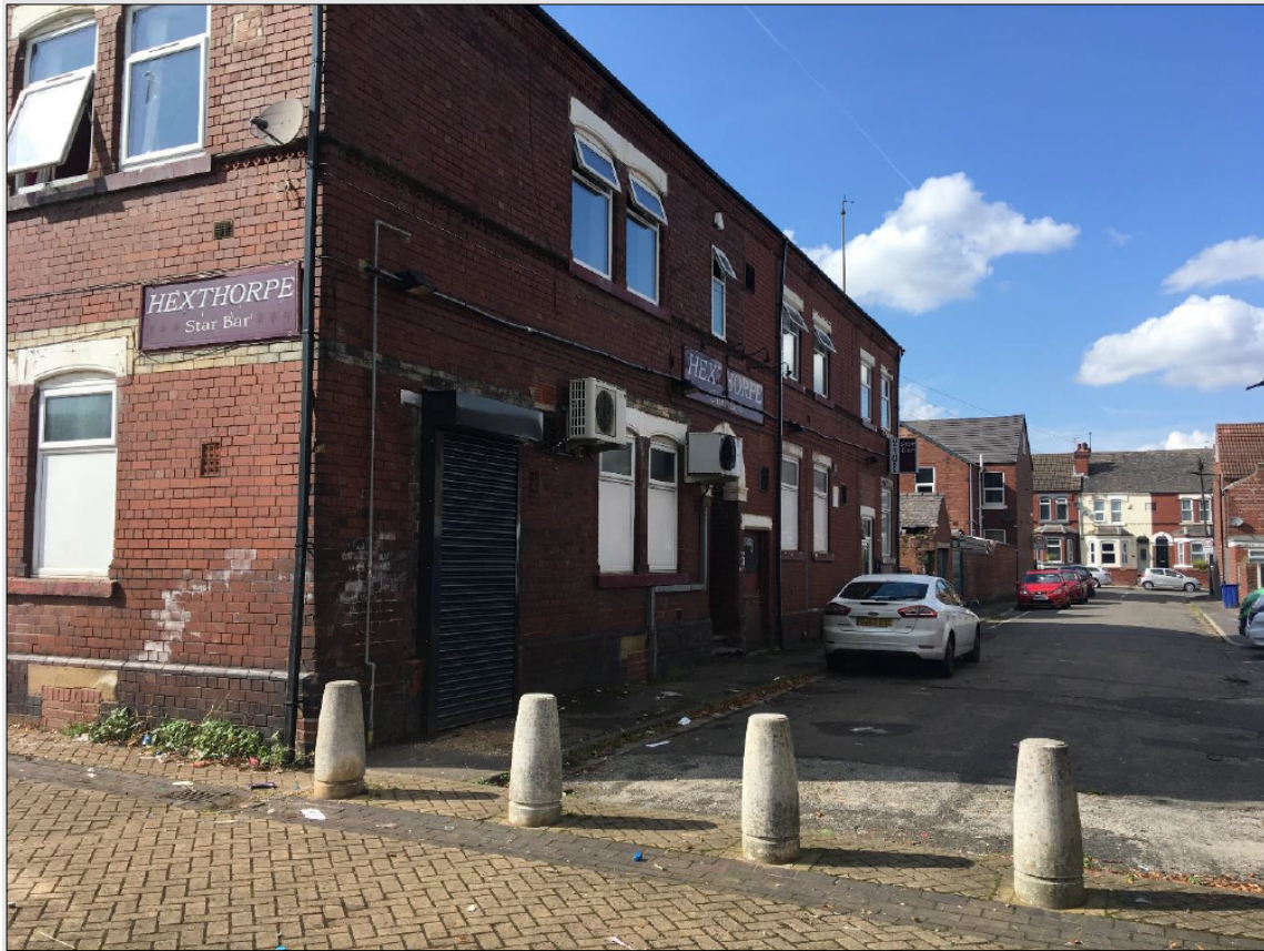
Photo 1: Application Site: Elevation at Langer Street
